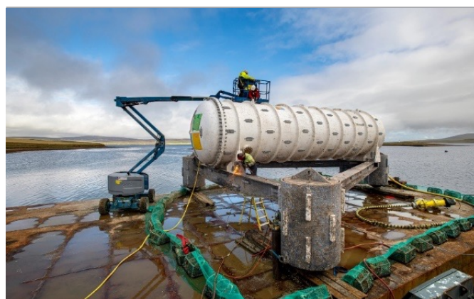
Figure 3: Microsoft's underwater datacentre 6 .
